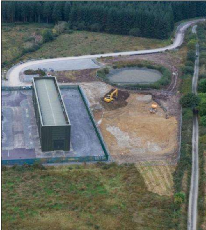
Plate 4-18 Typical 220kV GIS Switching Substation. Source: BnM
