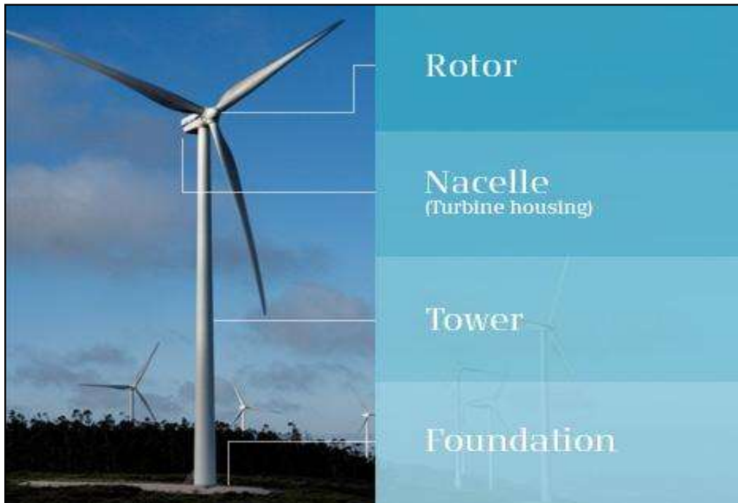
Plate 4-1 Wind Turbine Components
