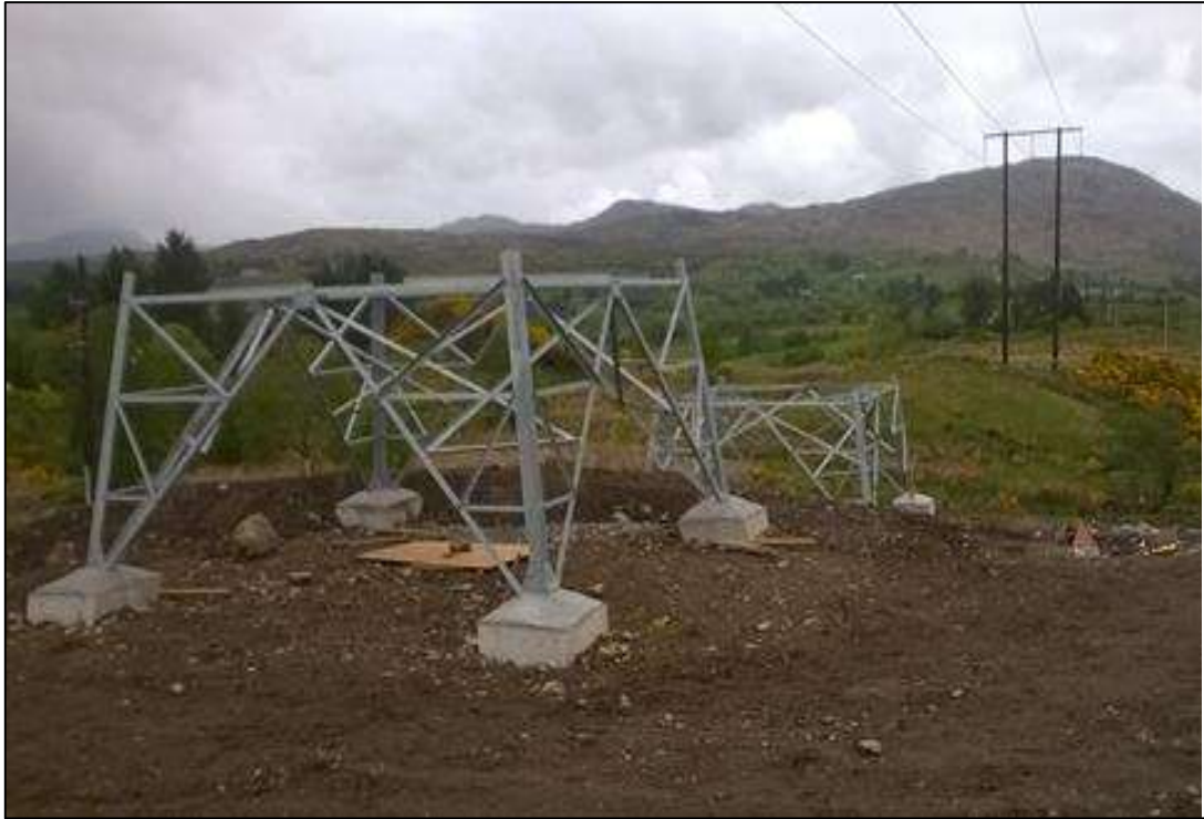
Plate 4-14 Steel lattice tower foundation complete. Source: BnM
