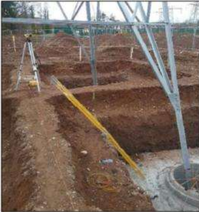
Plate 4-12 Steep Back Excavation. Source: BnM
