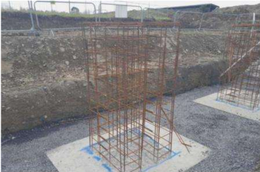
Plate 4-16 Stepped Back Excavation for Gantry Foundations. Source: BnM
