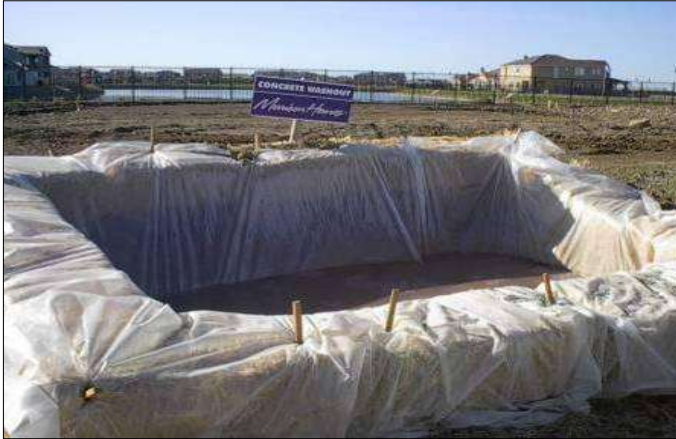
Plate 4-4 Concrete washout area
