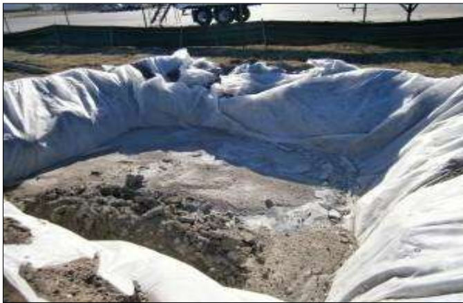
Plate 4-5 Concrete Wash Out Area
