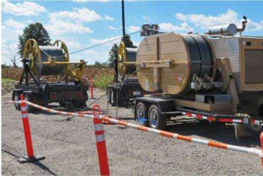
Plate 4-17 Puller – Tensioner Machine. Source: BnM
