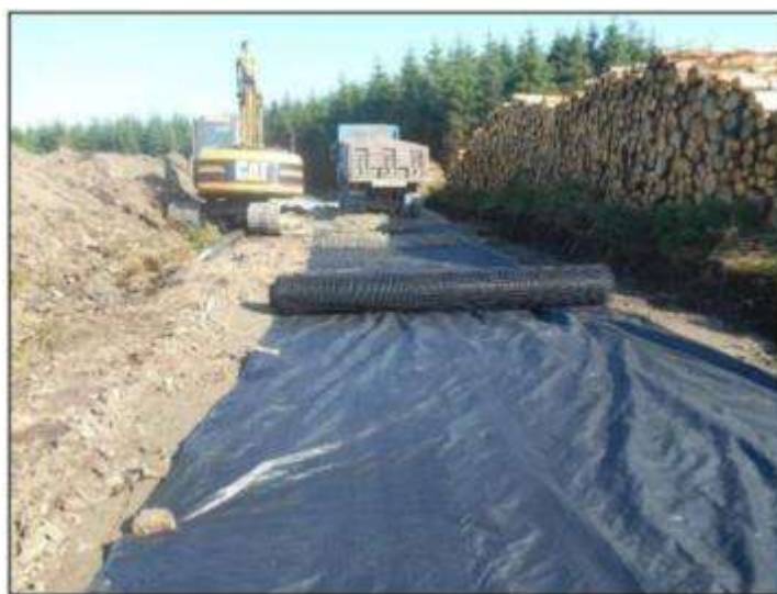
Plate 4-19 Crushed Rock Roadway Build-Up with Geo-Textile. Source: BnM
