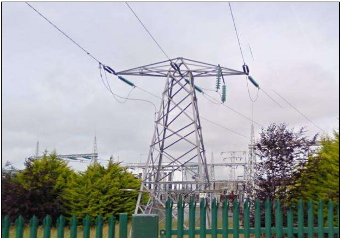
Plate 4-15 Completed End Mast Tower. Source: BnM
