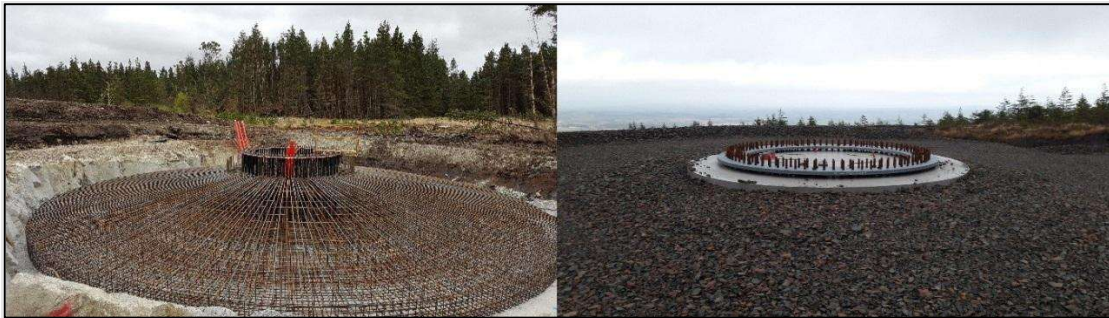
Plate 4-2 Turbine 'Anchor Cage' and finished turbine base
