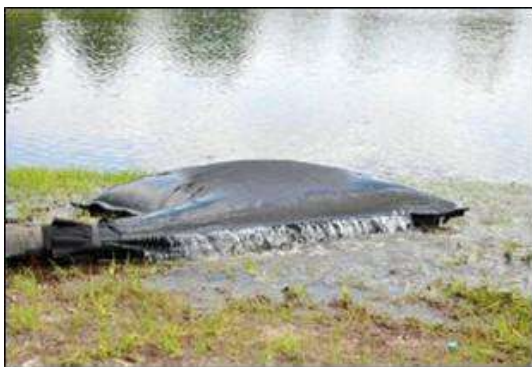
Plate 4-7 Silt Bag with water being pumped through
