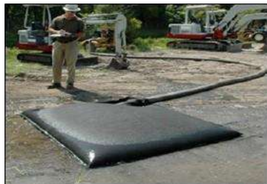
Plate 4-8 Silt bag under inspection
